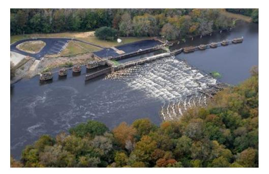
Figure 5 Existing Rock Arch Rapids Fish Ramp at Lock and Dam #1
